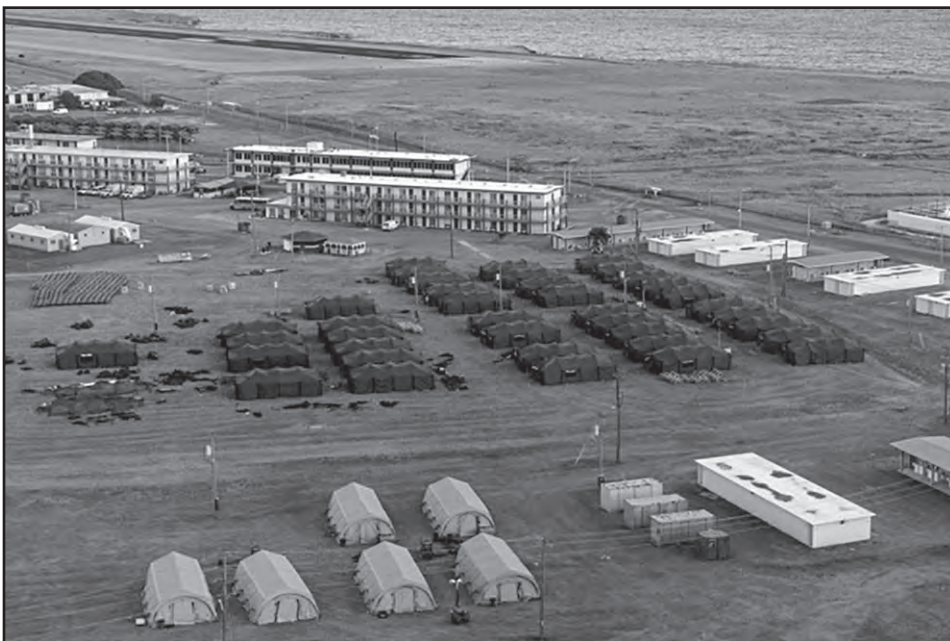
The new camp site where the Trump administration plans to house thousands of undocumented migrants at the U.S. naval base at Guantánamo Bay, Cuba.
